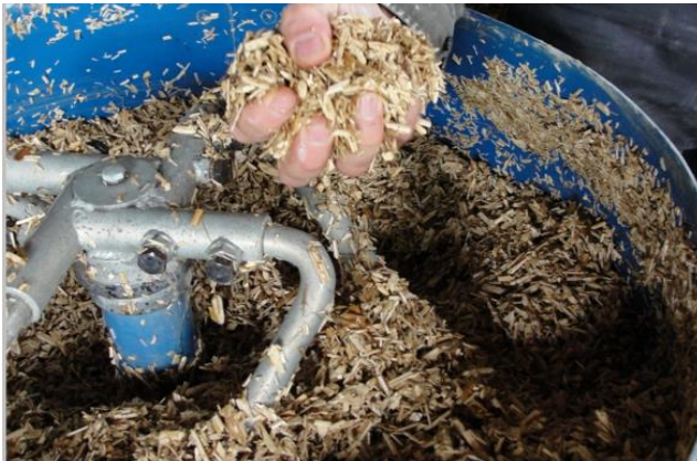
Figure 5: Hempcrete being prepared.
