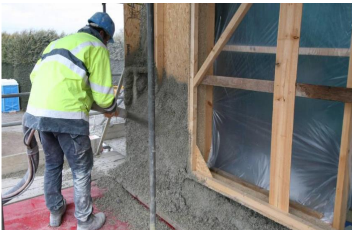
Figure 1312: Hempcrete Spraying
